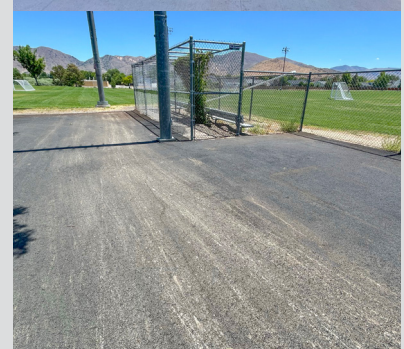
Mira Loma Park asphalt
